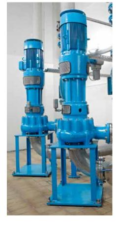
the modular system of our Turo® vortex pump. All types of design (submerged, dry mounted with vertical and horizontal configuration, close-coupled or bearing frame pumps, shaft or cantilever) are available.
